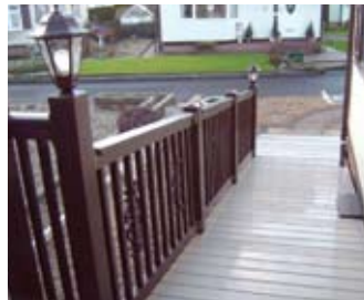
Wheelchair Ramp with Lighted Access
